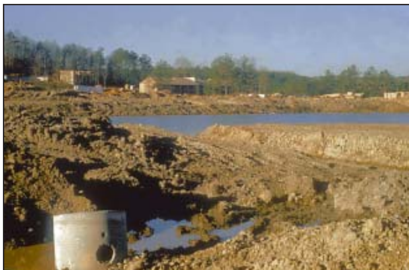
Figure 4.1 Development for housing has allowed erosion and sedimentation to occur which can affect the quality of nearby water.
