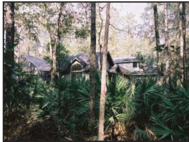
Florida retro-fit house BEFORE mitigation measures.
