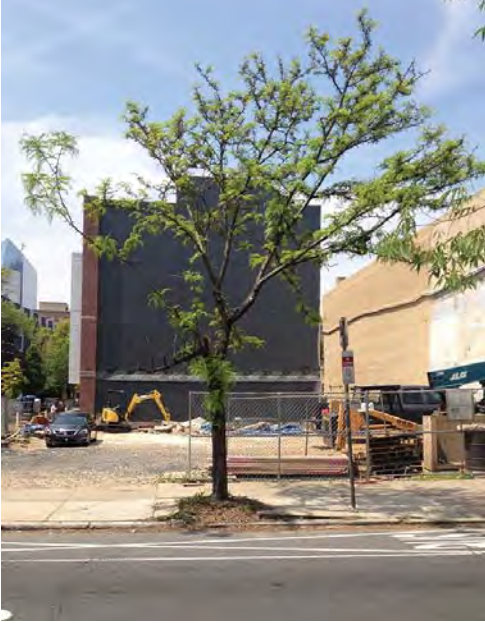
Site Type: Sidewalk Cut-out Land Use: Vacant Lot Photo: J.P. Fristensky
