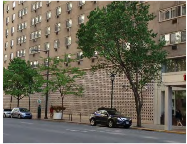
Site Type: Sidewalk Cut-out Land Use: Multi-family Residential Photo: L.A. Roman
