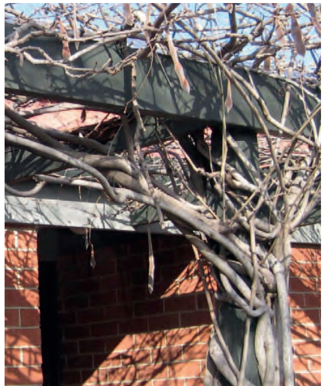
Vines and creepers act as ladder fuels.
