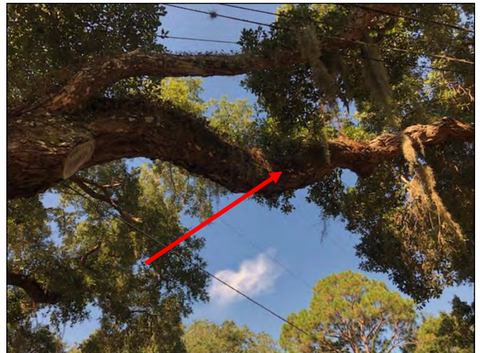
Live Oak with a Decayed Limb Over the Road, Needs Pruning
