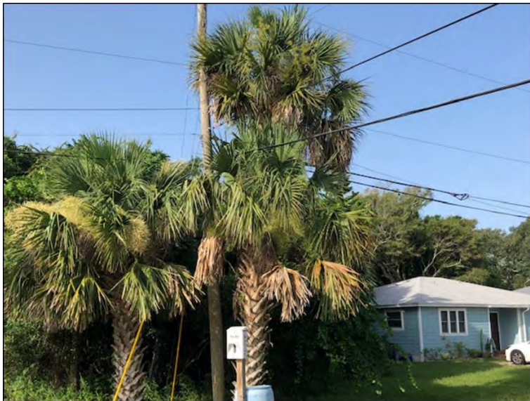
Palm Tree Embedded in the Wires and Conductors
