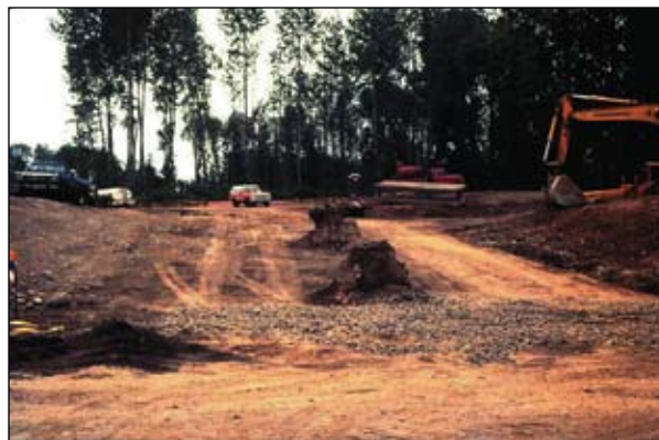
Figure 7. Stripping of topsoil during construction removes most of the nutrients and organic matter vital to plant growth (Source: Derek Booth)
