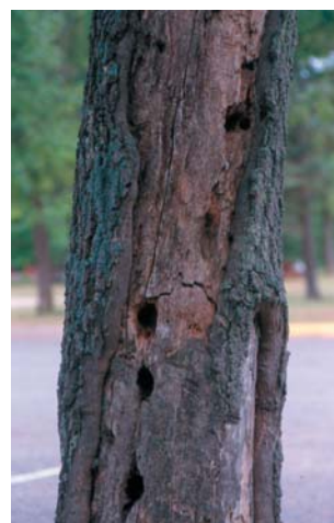
Figure 3.64. Horizontal cracks are rarely found because they develop just before trees fail.
