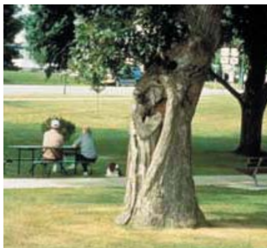
Figure 5.28. This tree has a very large wound that was created when a large branch was previously removed.
