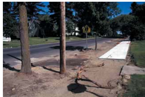
Figures 3.91-3.94. Roots are often removed or damaged during construction.
