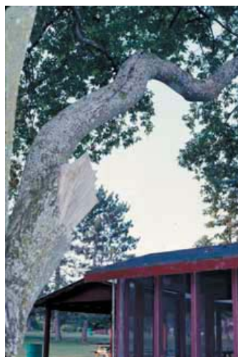
Figure 3.69. High risk of failure: When any large branch is cracked.
