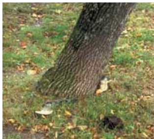
Figure 3.81. A leaning tree that also had advanced decay in the root collar.
