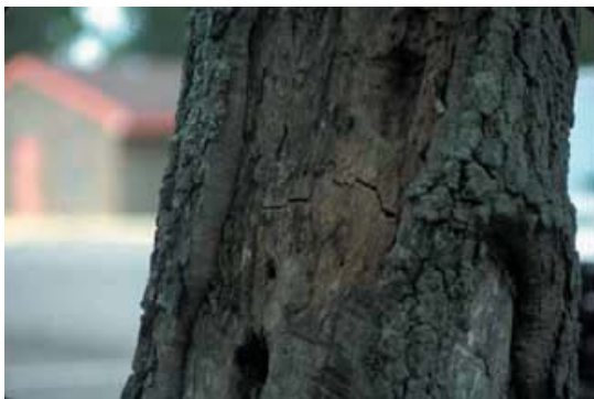
Figure 3.139. Tension symptom: Horizontal crack in wood of leaning tree.
