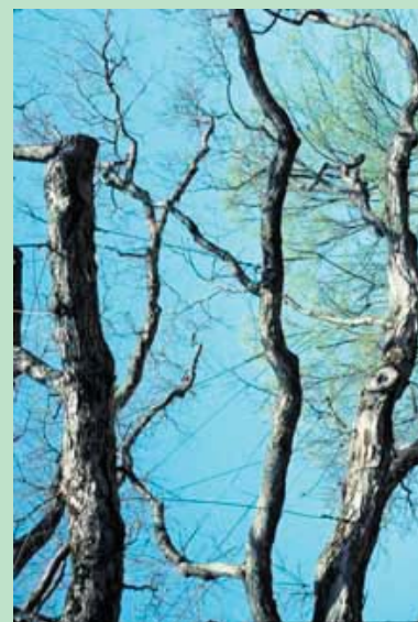
Figure 5.16. In this leaf-off view, some slack can be seen in the cables due to the reduced weight of the branches.
