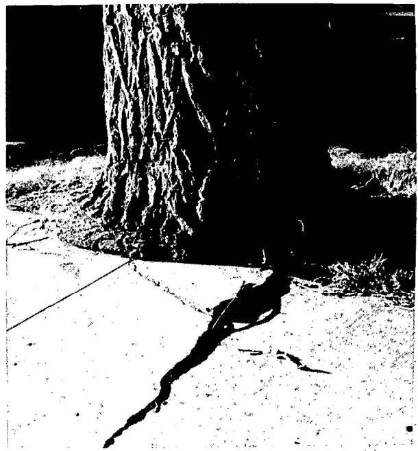
Figure 7-1. Trees planted too close to sidewalks— or sidewalks constructed too close to trees— cause premature sidewalk failure which threatens the safety of citizens
