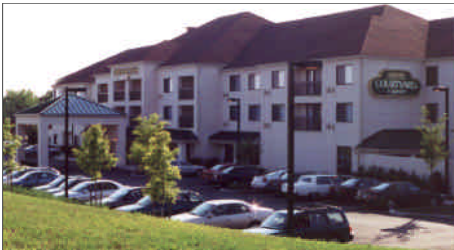
Bermed hillside adjacent to highway buffered roadway noise and provided better views from hotel rooms looking outward.
