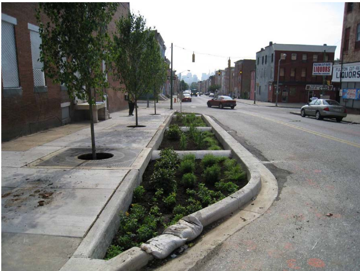
Figure 6. Example using trees and bioretention in Baltimore, MD. Source: City of Baltimore.
