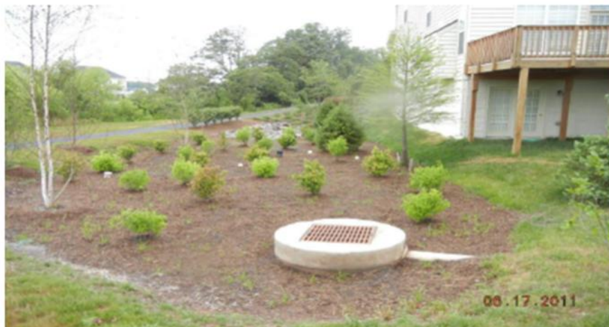
Figure 4. Trees planted within a bioretention facility. Courtesy of Boyd Church in Loudoun County, Virginia.
