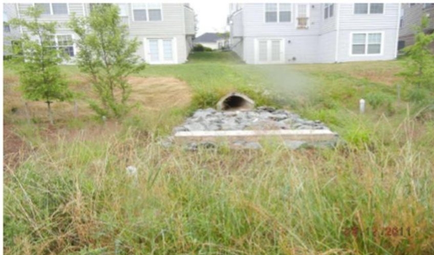
Figure 3. Trees (River Birch) planted within a bioretention facility. Switchgrass vegetation is also present. Courtesy of Boyd Church in Loudoun County, Virginia.
