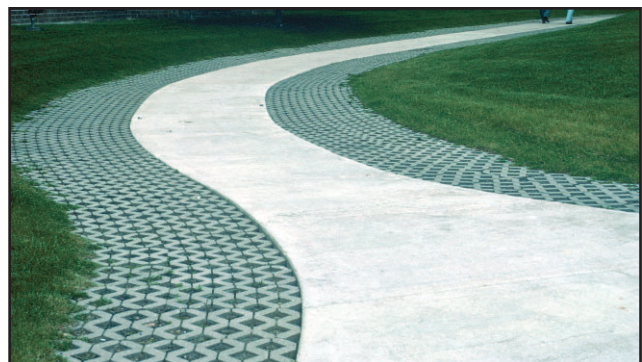
To reduce de-icing salt damage, open pavers have replaced turf along the sidewalk edge.
