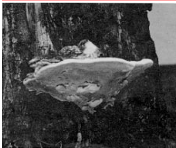
Figure 8. Fungal fruiting structures called conks indicate the presence of wood decay.
