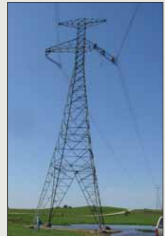
230-kV/345-kV lattice transmission structure
