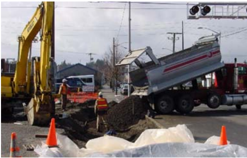
Dump truck, dumping load of structural soil into excavated area. Engineer determined dumping and spreading sufficient to reach 85% design compaction.
