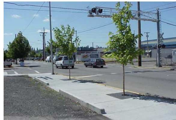
Trees installed in structural soil, South Side of State Avenue, looking West
