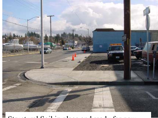
Structural Soil in place and ready for new trees.
