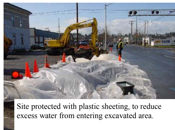
Sidewalk demolished, and existing soil being excavated.
