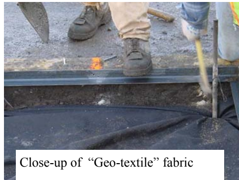
Project site, looking East, showing, structural soil in place and forming for new curb on corner of State and Jefferson.
