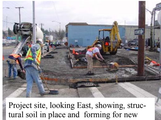
First lift of "structural soil" being compacted, later determined to be unnecessary.
