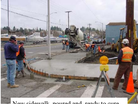
New sidewalk, poured and ready to cure.
