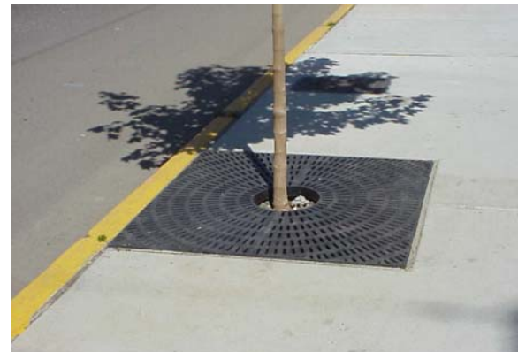
Close-up of tree planted in structural soil, with a plastic tree grate installed.
