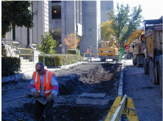
Typical structural soil streetscape installation (above). Trees growing in structural soil in high-use area (below). Photos courtesy of Dr. Nina Bassuk, Cornell University.
