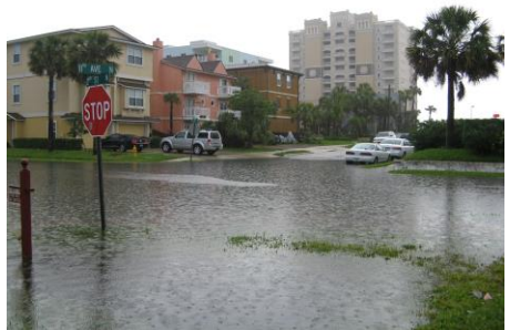
Stormwater is a problem for cities across the country. Existing grey and green stormwater management systems are often not enough to accommodate runoff. Adding trees to those systems is a cost-effective way to improve their function and reduce runoff. Photo courtesy of Davey Resource Group.
