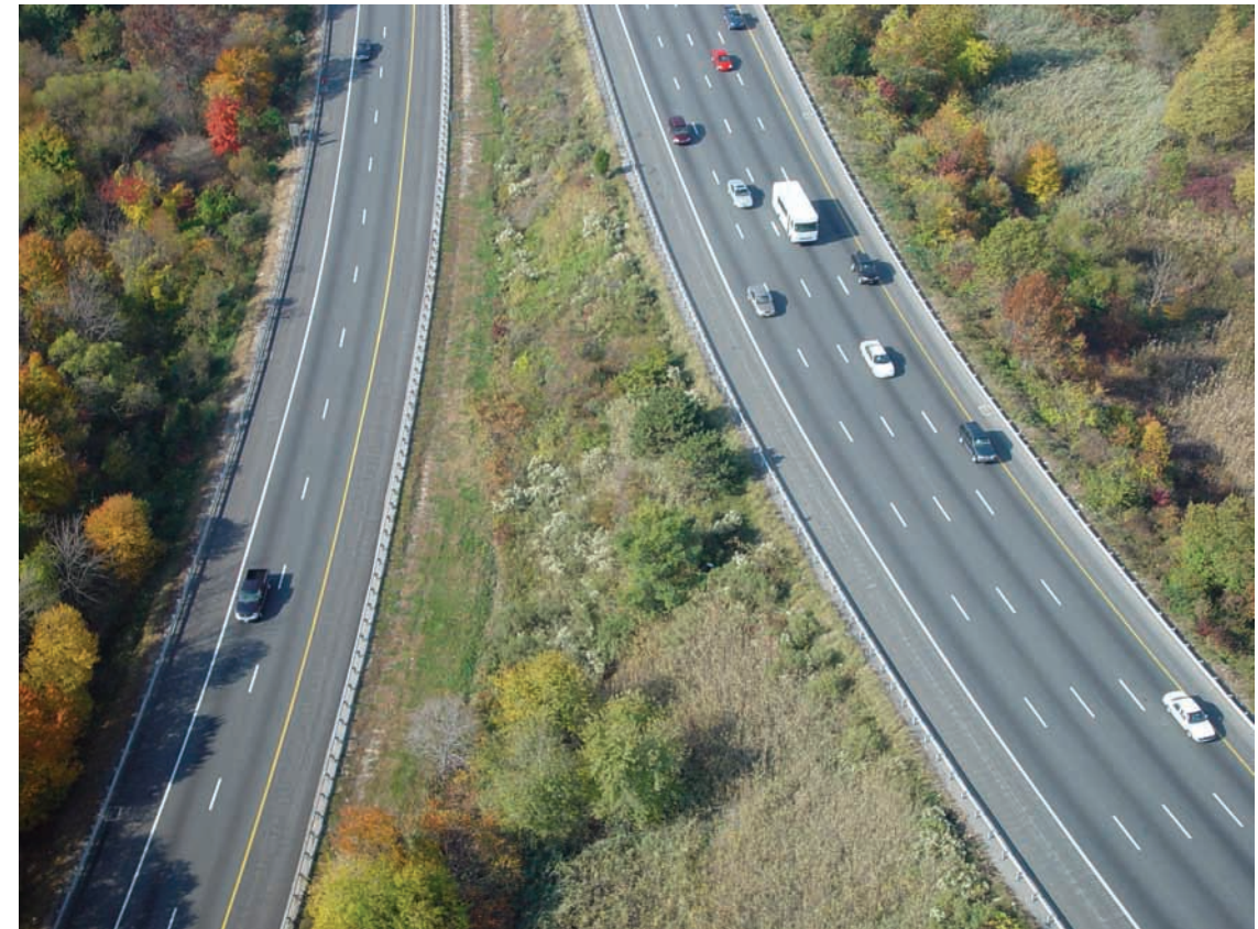
Continuity of roadside and median vegetation immerses the traveler in the patterns and colors of the regional landscape.
