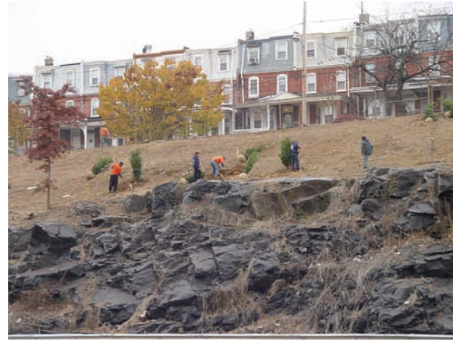
Eastern red cedars are planted in a naturalistic arrangement along the dry, rocky I95 cut through Wilmington. Requiring less supplemental water than bare root or container material during establishment, balled and burlapped trees offer the best chance of survival in this challenging environment.
