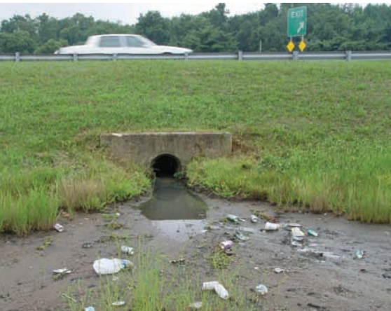
Pollutants in the runoff at this outflow from I-95 are an example of the extreme conditions faced when trying to revegetate the roadside environment.
