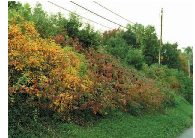
Trees can be treated as cutbacks too. Stabilizing a slope along Route 896, this mass of sassafras and sumac results from periodic cutting back, brightening the autumn roadside with complementary colors.
