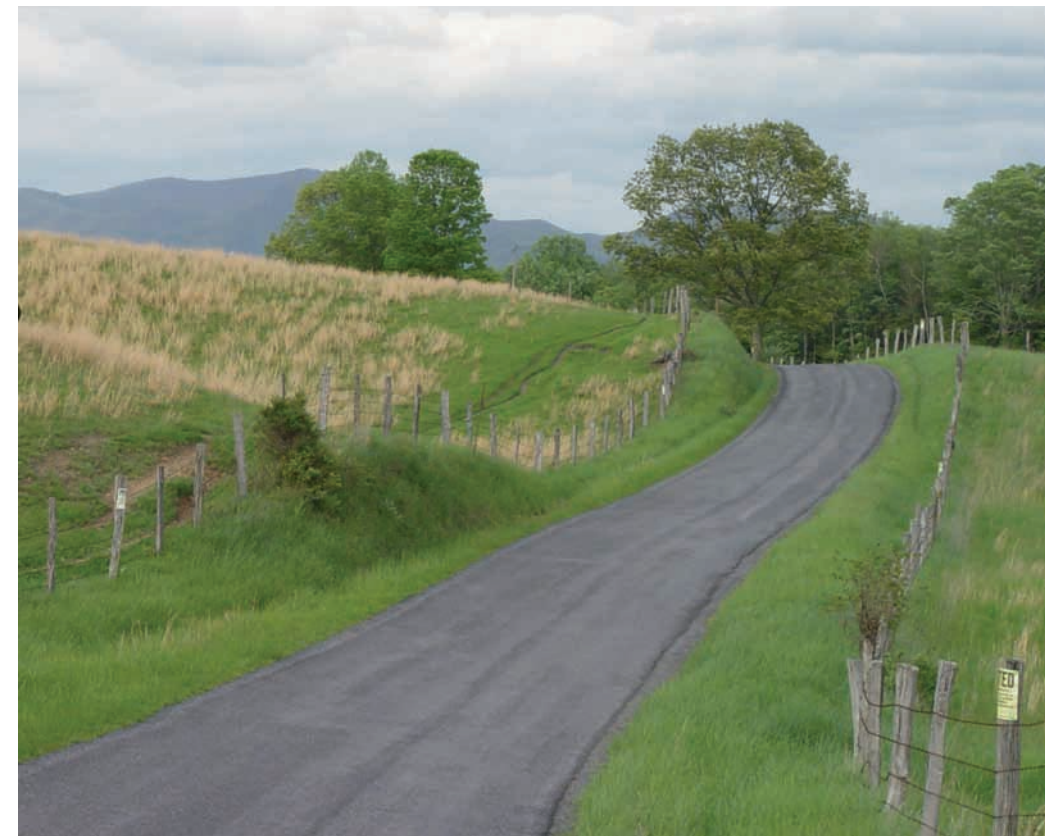
Trees visible beyond the crest of the hill help drivers anticipate an upcoming turn to the left.
