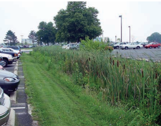
Vegetation in this parking lot swale slows runoff and increases infiltration.
