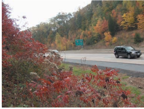
An established colony of sumac holds the slope and creates sufficient shade within its spread to discourage weed competition.
