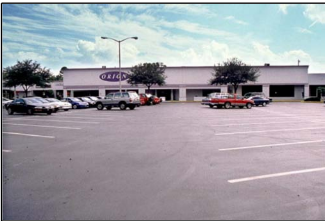
Figure 18. The urban forest ecosystem through evaporative cooling and shade can contribute to reducing the temperatures in the urban heat island. This parking lot is a contributor to high temperatures in the urban heat island.
