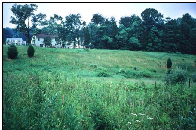
Figure 49. Zone 3 is a flat grassy area about 10m wide at the urban/buffer interface. Its major function is to convert channelized urban flow into sheet flow and slow water velocity to less than 0.3 m/sec. Zone 3 performs some settling, filtering, and infiltration. Photos are of the "Difficult Run" urban riparian project, courtesy of Judy Okay, Virginia Department of Forestry.
