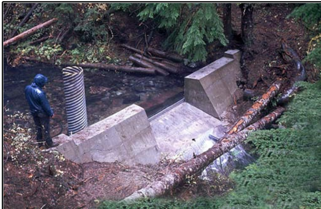
Figure 14. A weir is one type of structure used for measuring forest stream flow. It is an important tool for answering questions about the effects of land management on the hydrological cycle. Photo by Hans Riekerk.
