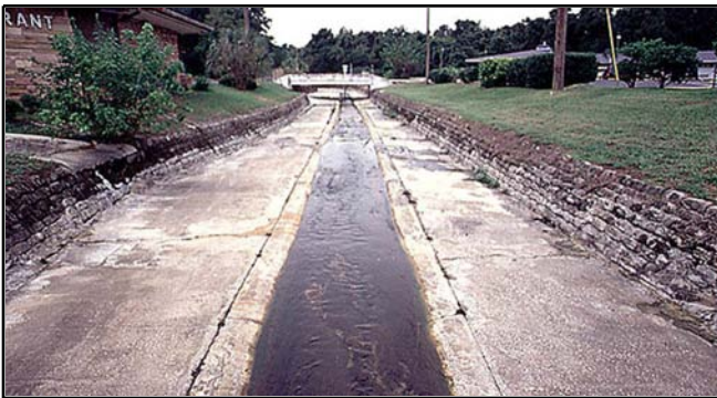
Figure 58. Even with the best of water quality this urbanized stream will be a non-functioning ecosystem. The stream morphology has been altered, the bottom substrate paved over, and stream communities have been eliminated.
