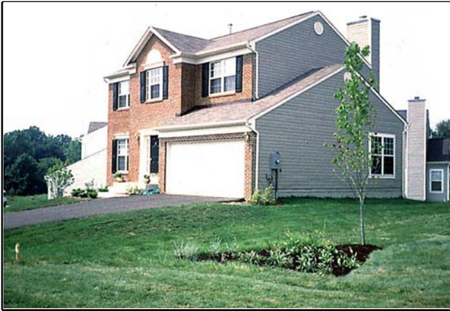
Figure 57. Large stormwater treatment facilities often have poor pollutant reduction performance. A better solution is to keep stormwater on site and allow it to be filtered by the soil. This picture shows a "rain garden" where runoff from the roof and driveway will be retained and pollutants filtered out by the soil. Photo by Judy Okay, Virginia Department of Forestry.
