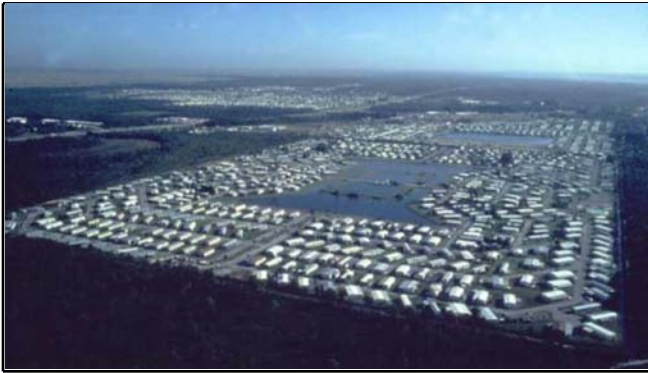
Figure 19. Most species of birds, mammals, reptiles and amphibians feed or breed in wetlands but also need access to surrounding uplands to fulfill all of their life-sustaining requirements. This wetland, for instance, has no upland connection.
