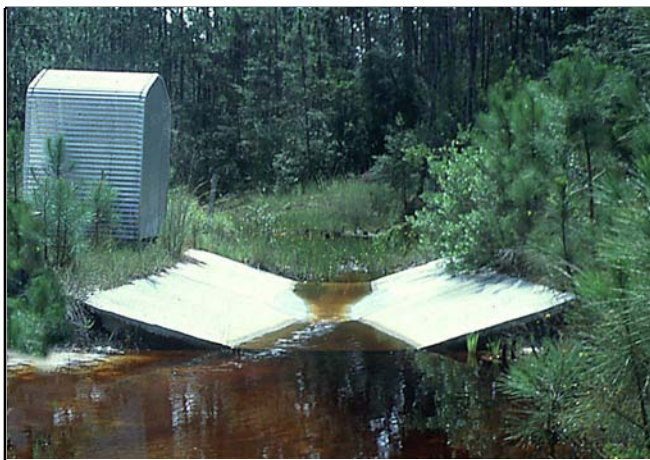
Figure 36. Flumes are flow modification structures designed to accurately measure the amount of water passing through them. They are self cleaning and can work with relatively low head loss, but they are very expensive.
