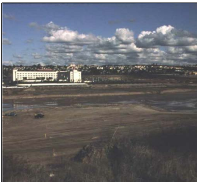
Figure 2.1 Photo by John Rieger, CA Department of Transportation
