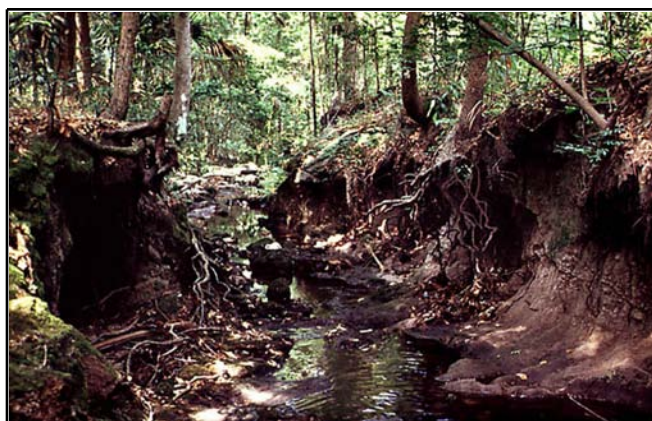
Figure 30. High energy urban stormwater runoff scours stream bottoms, erodes and undercuts their banks. This degrades aquatic habitat and creates dangerous landslide conditions.
