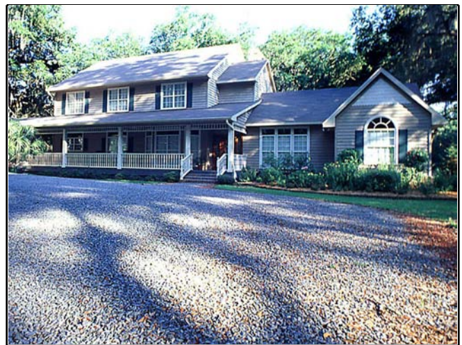
Figure 56. Reducing the impervious surfaces at a home by having an attractive gravel driveway instead of an impervious paved one, will significantly reduce the amount of water and pollutants that runoff property. The cumulative impact of many citizens reducing their pollutant load can make the restoration of aquatic ecosystems possible.
