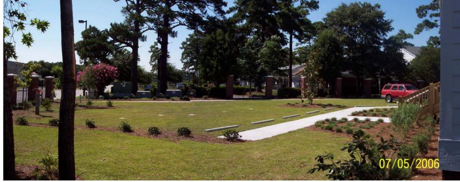
The parking lot utilizes grass pavers created by *Invisible Structures* combining the qualities of grass landscaping with the durability of a paved parking lot. Stormwater runoff and the heat island effect created by impervious surfaces was eliminated.
