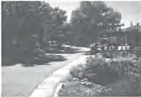
Bioswales alongside streets can filter and infiltrate street runoff. This swale is at Village Homes in Davis, California.
