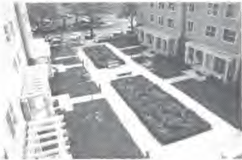
Stormwater planters at Buckman Heights Apartments in Portland, Oregon collect runoff from roofs and the plaza for up to five year storm events. Over flow is directed to drywalls.
