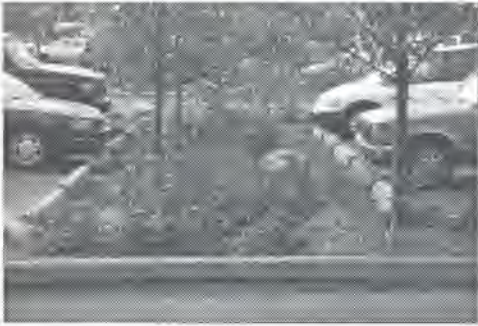
By reversing the curvature of planted "islands" in parking lots, these landscape strips become filters and infiltration zones for parking lot runoff. These biofilters at the Oregon Museum of Science and Industry are estimated to filter 90% of the pollutants from runoff.
