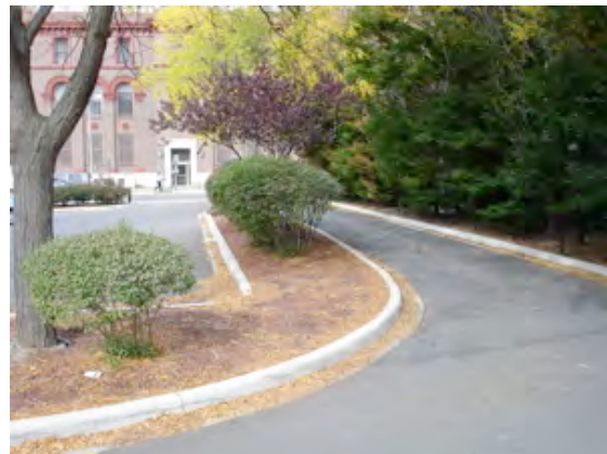
Within a parking lot, raised areas can define the ends of parking aisles, marking driving lanes. Using nature in this way is more visible than lines painted on the ground. These features can increase both clarity and safety of all who use the space.
