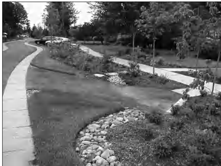
Green engineering, which increases water infiltration into soils, reduces stormwater and makes places more attractive.
