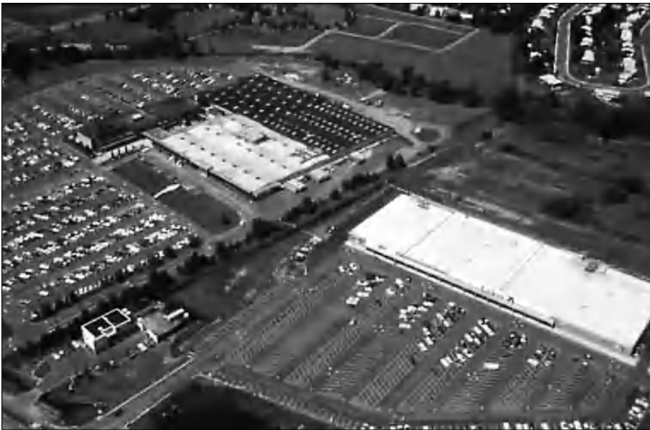
The large impermeable surfaces of parking lots and roofs cause large stormwater management costs.
