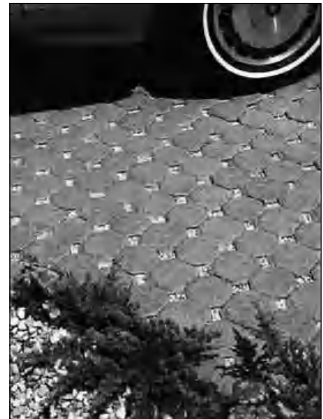
The green engineering of bioretention areas and permeable paving can be used to increase water infiltration, increase water quality, and decrease stormwater costs.
