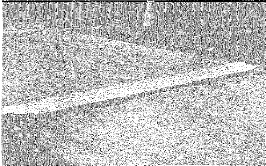
Figure 2. Mechanical grinding
