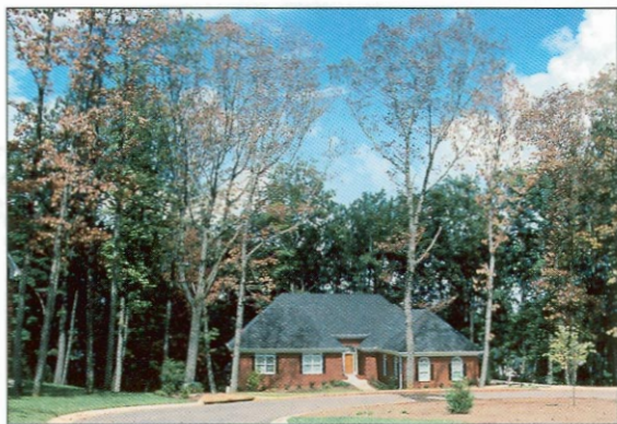
Figure 1.--Trees stressed by construction damage.
