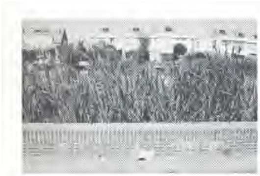
At Ecolonia, The Netherlands, street runoff passes through a mouse hole to dense wetland plants on its way to a stormwater pond that is the central feature of the community.
