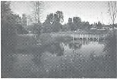
Meadowbrook Pond in Seattle, Washington, is a flood diversion pond and public park constructed to save a salmon run.
