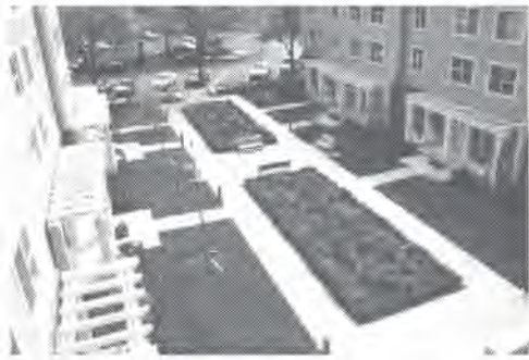
Stormwater planters at Buckman Heights Apartments in Portland, Oregon collect runoff from roofs and the plaza for up to five year storm events. Over flow is directed to drywalls.
