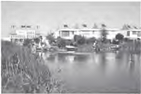
This large stormwater treatment pond at Ecolonja, The Netherlands is the central landscape feature of the community.
