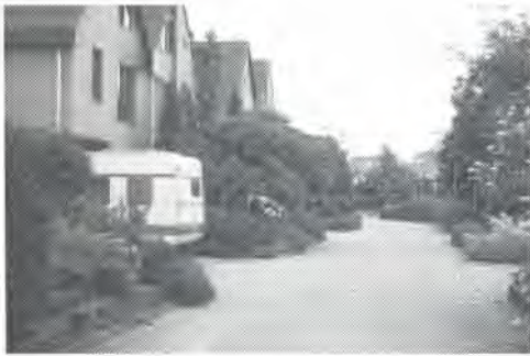
A very narrow access road in Houten, The Netherlands, provides a safe, attractive street environment, while drastically reducing paved area.
