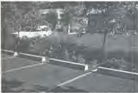
Biofiltration swales replace conventional traffic islands in a Portland, Oregon parking lot. These swales are found to be 90% effective at removing pollutants associated with vehicular areas (Bureau of Environmental Services, 1999)
