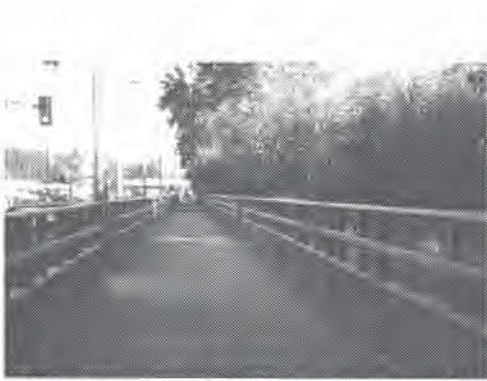
Bridging a wetland adjacent to a commercial district in Bellevue, Washington
