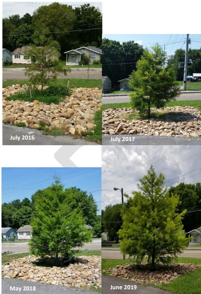
Figure 13 Baldcypress tree growing in gravel bed stormwater retention system from 2016 to 2019
