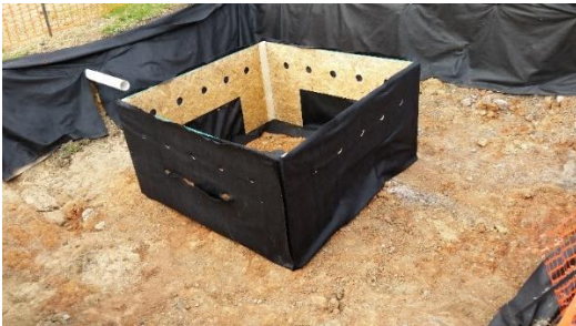
Figure 5 Mineral soil bed form was covered with an 8 ounce non-woven geotextile fabric to provide additional separation support of mineral soil and gravel after the OSB form disintegrates. Slits were cut into the fabric to allow roots to migrate from the mineral soil into the gravel layer.
