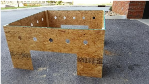
Figure 4 A wooden form constructed of 7/16" Oriented Strand Board (OSB) was used to keep the mineral soil separate from the gravel layer.
