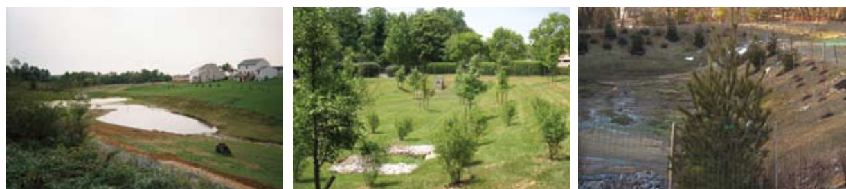
Figure 17. Storm water ponds with trees incorporated offer benefits over a conventional storm water pond with no trees (left).
