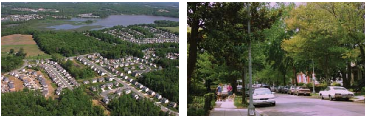
Figure 1. Large tracts of forest (left) and mature trees (right) can be conserved during development. Photos: Left—Maryland Department of Natural Resources; Right—District of Columbia Department of Forestry
