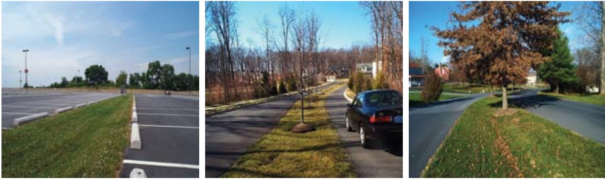
Figure 18. Swales with trees offer greater benefits than a swale with no trees (left).
