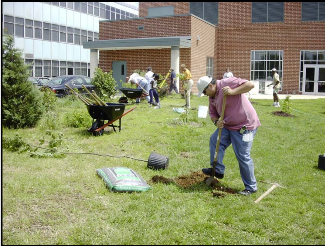
Figure 27. Amending soil with compost at a planting hole
