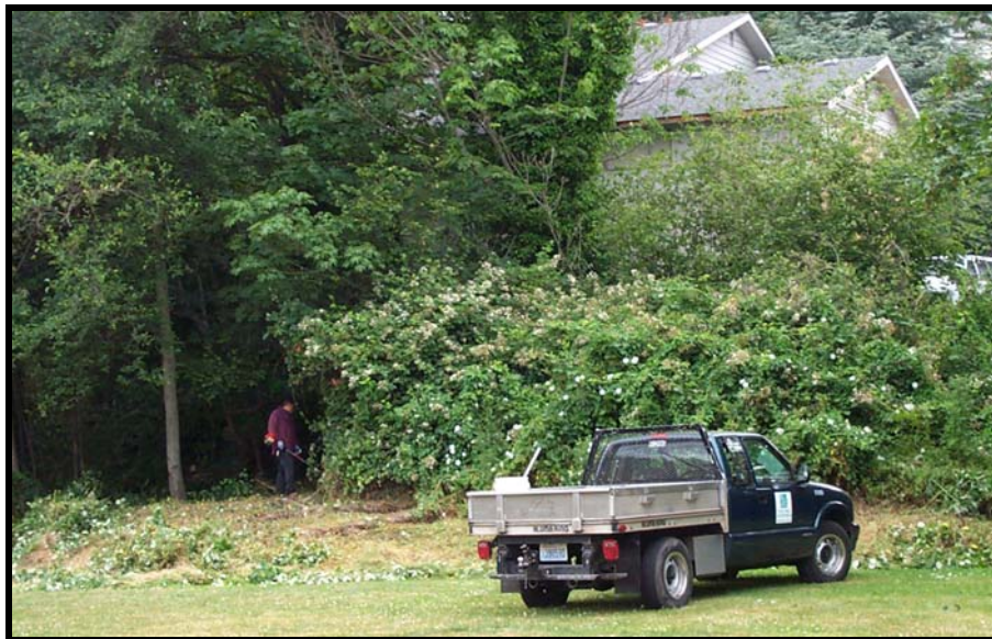
Figure 25. Removal of invasive species using a chainsaw
