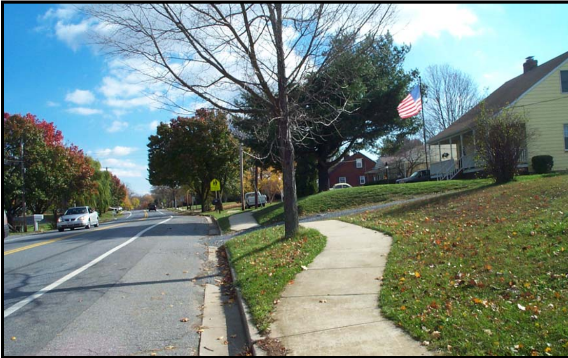
Figure 17. Curving sidewalk allows space for street trees
