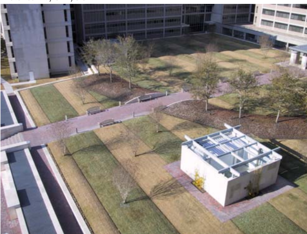
A green roof on the Baylor Research Institute in the Texas Medical Center provides intensive planting on top of this large structure.
