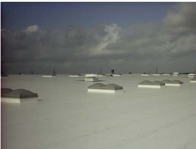
Reflective roofing application in Houston.
