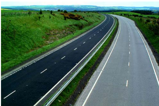
This photo simulates a conventional asphalt overlay on the left with asphalt lightened by color additives on the right.
