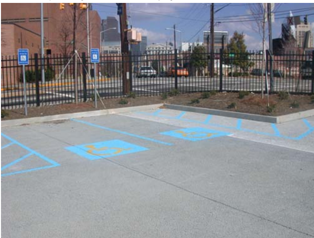
Example of porous concrete used on parking lot in Atlanta. Note that there are various porous concrete and paving options, available for a wide range of applications.
