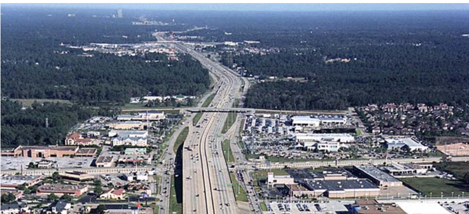
Urban development can involve removal of most of the existing tree canopy, as shown here on I-45 in a heavily forested area. Conservation measures are particularly important in such locations.
