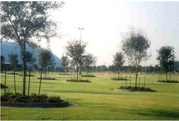
GrassPave application shown in the top photo, and the finished product, a grass and tree covered parking lot at Reliant Park (below) in Houston.
