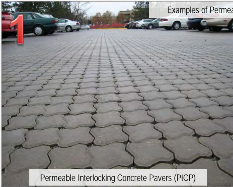
Permeable Interlocking Concrete Pavers (PICP)
