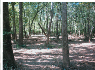
Understory after GyroTrac mulcher.
