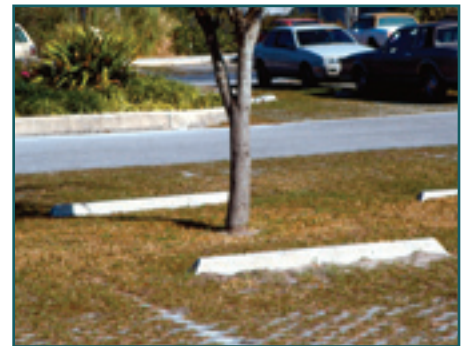
Consider soil properties (soil depth, water table and compaction). This porous surface reduces runoff and improves root health.
