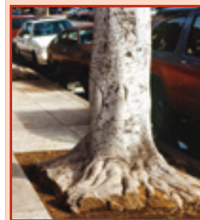
Hazard: major support roots cut.
