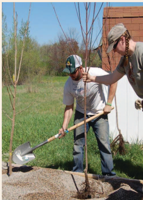
Figure 11 (above). Installing trees in gravel bed with shovel.
