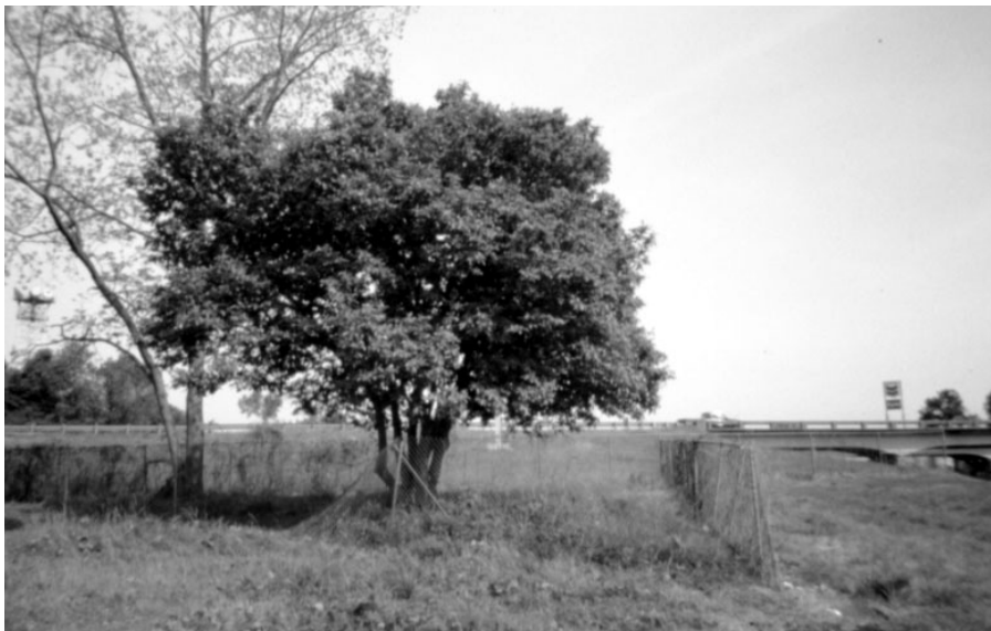
Protect roots from compaction by erecting barriers around or slightly beyond the dripline of trees during construction.
