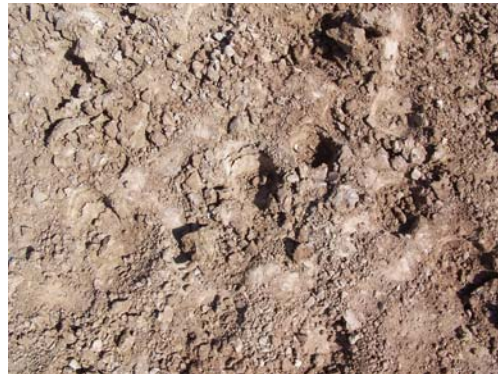
Figure 5.3: Sheepsfoot rollers compact soil.
