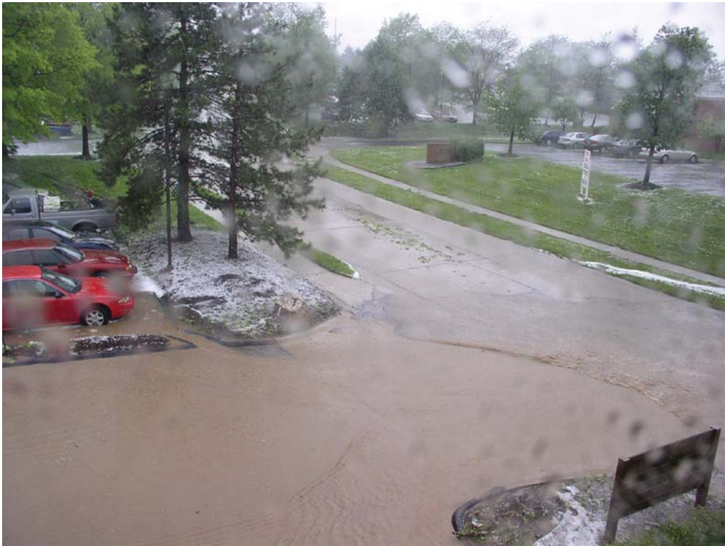
Figure 3.12: A flooded parking lot and street.
