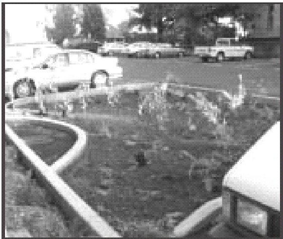
Parking lot rain garden (from PSAT 2003)
