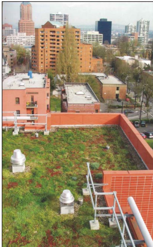
Figure 1-4. Example of a living roof. Hamilton City Apartments, Portland OR. Source: Environmental Services of Portland Brochure.
