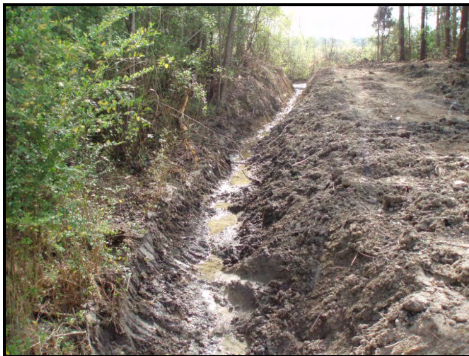
Figure 8. This South Carolina wetland was being drained and ditched in July 2006.
