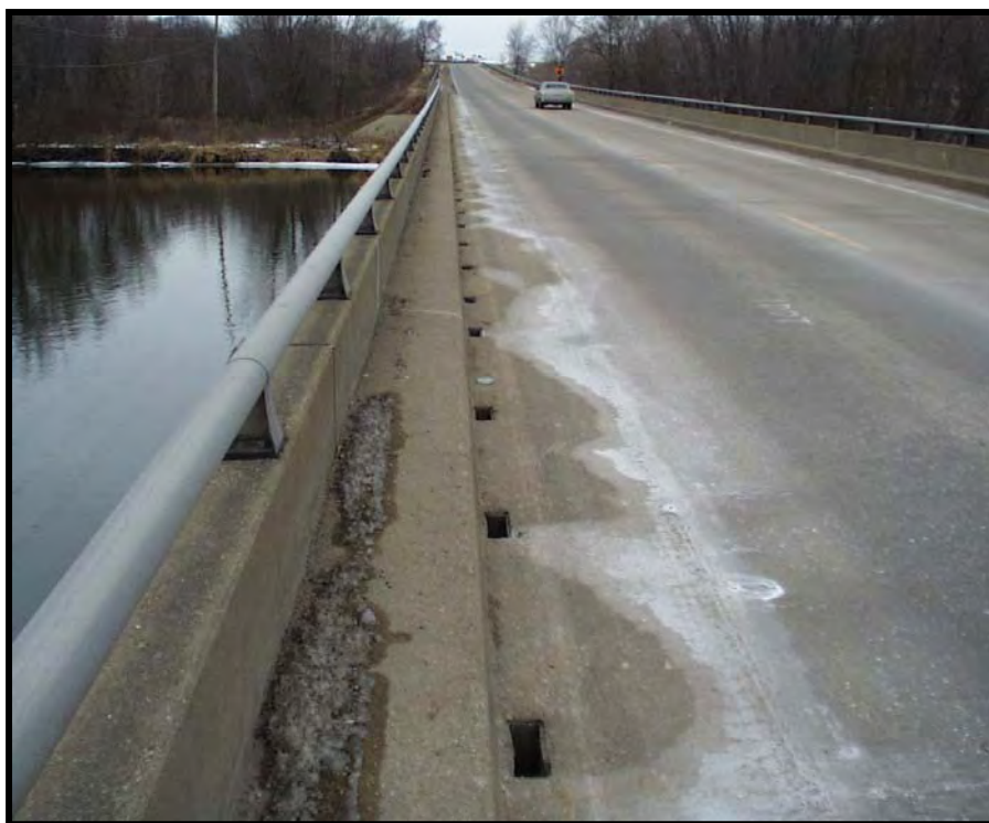
Figure 18. Road salt is a major source of chloride to surface waters (Source: Beloit College)
