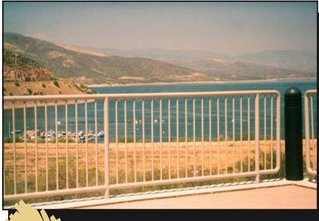
Figure 79—This railing is safe, meets code requirements, and provides a great view, even when you look through the rails.
