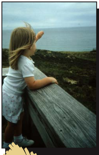
Figure 80—Caution: railings with horizontal rails make an inviting ladder for small children.
