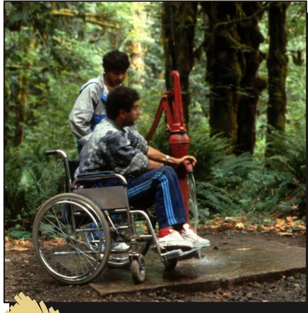
Figure 12—Others used to have to do the pumping.
