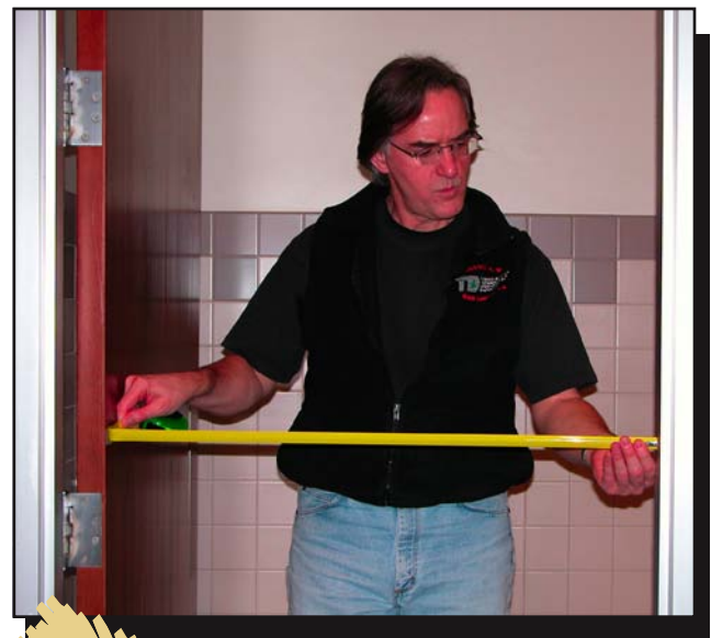
Figure 10—All doorways must have a minimum of 32 inches (813 millimeters) clear width.
