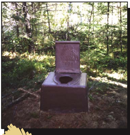
Figure 84—A fiberglass riser for a pit toilet in the Boundary Waters Canoe Area.
