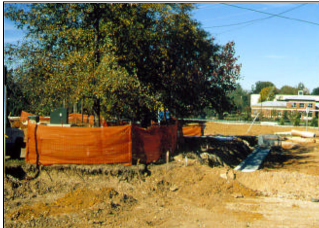
Figure 10 Even a minimal Tree Protection Zone (this one is substandard) during construction can significantly affect the survival of mature trees during human landscape change.
