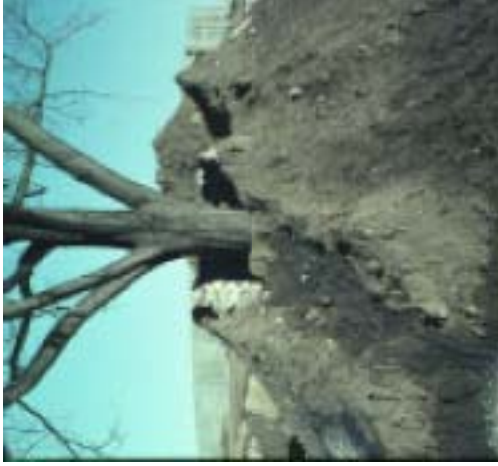
Figure 21. Parking equipment (a) or storing soil (b) within the protected root zone cause soil compaction and affect tree growth and survival.
