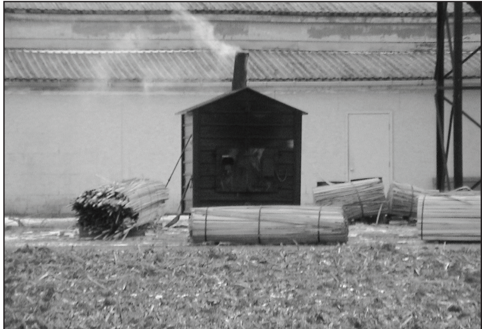
Figure 1. Outdoor boilers heat water that warms nearby buildings. PHOTO BY PHILLIP BADGER.
