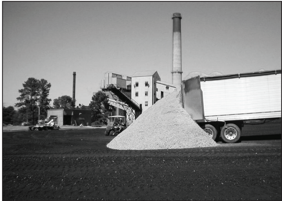
Figure 1. The Plant Gadsden uses coal, wood chips, sawdust, and switchgrass. PHOTO COURTESY OF SOUTHERN COMPANY.
