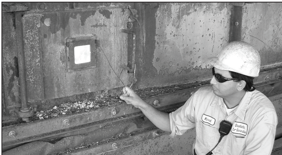
Figure 2. The Okeelanta Cogeneration Facility also burns invasive exotic melaleuca trees for fuel. PHOTO BY MARTHA C. MONROE.
