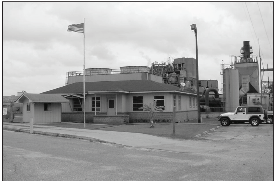
Figure 1. Telogia Power, LLC produces up to 14 MW of electrical energy each hour.
